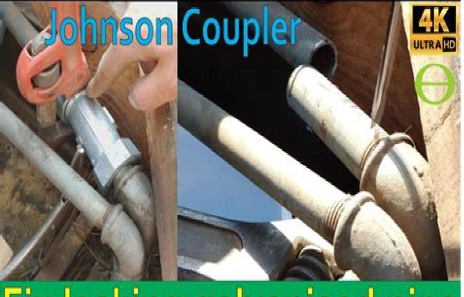
Fix leaking galvanised pipe
