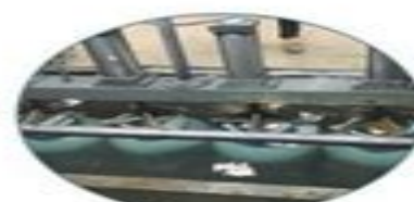
Air leakage testing
