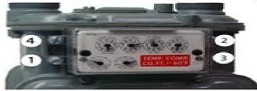
Examine the mounting screws. If they are 5/8-inch long and not corroded, keep them to re-attach the 100G DLS assembly. If the screws are not the correct length or if the screws are corroded, discard.
