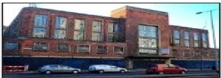
'A BLIGHT' The former John Lewis department store in Hull city centre. (Picture: Peter Harrison)
