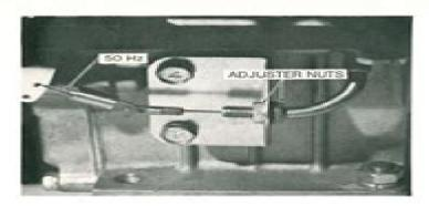
In order to produce alternating current at the correct frequency (60 Hz or 50 Hz), the engine must run at the correct speed, which is controlled by the governor. To adjust running speed:
