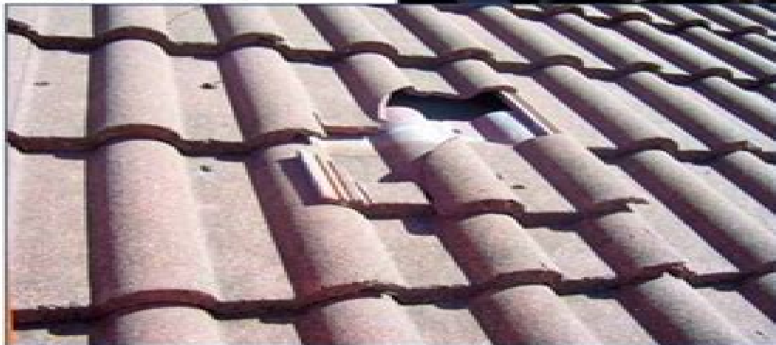
Photo 6 – Damage to concrete tile.
