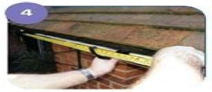
Mark the position of the fascia brackets, spacing them no more than 800mm apart (600mm in areas of heavy snowfall) and no more than 150mm from any angle or stopend.
