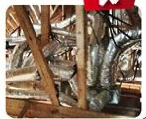
This improperly installed Flex Ductwork is a heart attack waiting to happen. The HVAC unit will not last as long as it should and this type of Flex Duct install will increase energy consumption.
