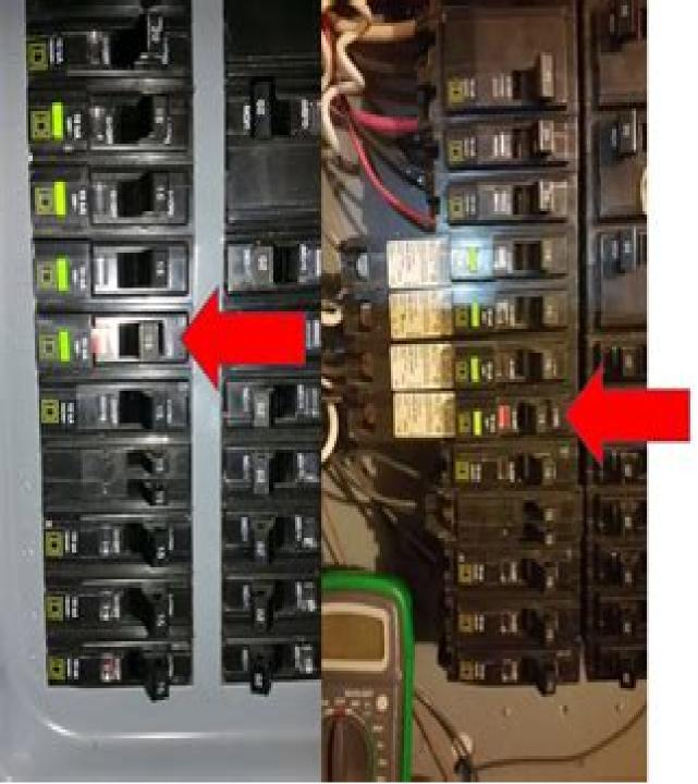
This type of circuit breaker is a GFCI with intermediate trip position (see the RED tag from the transparent window)
