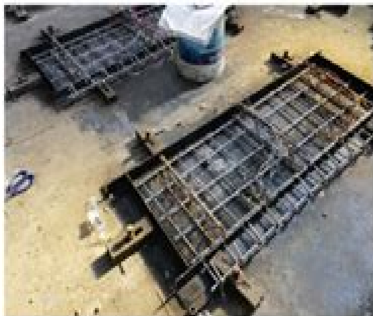
(a) precast slab production
