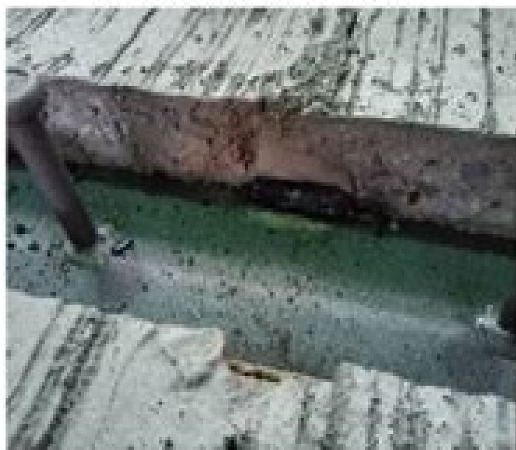
(c) welded angle
