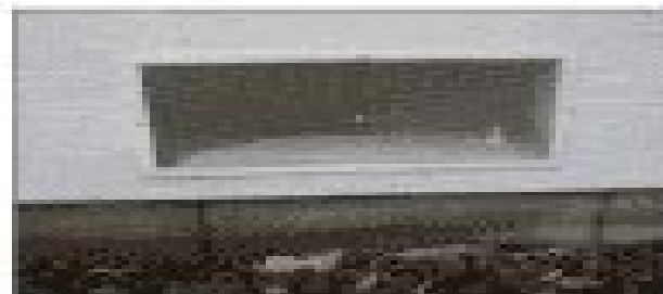
Figure 1. A closed foundation with a cripple wall (FEMA for all seasons)
