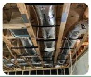
The air distribution network (ductwork) is like the arteries in the body that's connected to the heart. The Flex Ductwork is connected to the HVAC unit. If the ductwork (arteries) are not correct, then the heart (HVAC unit) will fail permanently.
