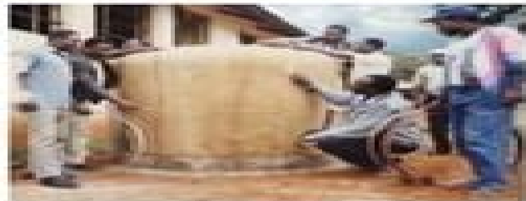
Figure 2-15: Place the joined jute cloth-covered jar mould onto the foundation.
