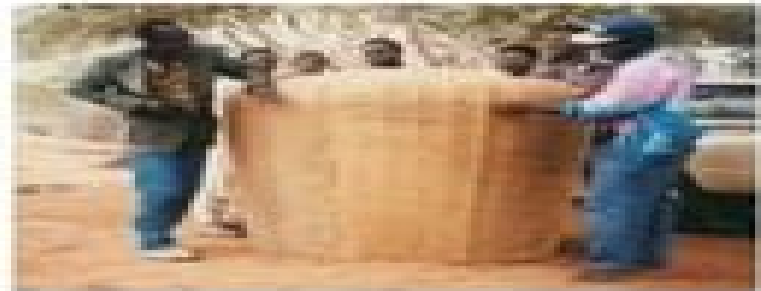
Figure 2-14: Join the jute cloth-covered segment moulds together with binding wire.
