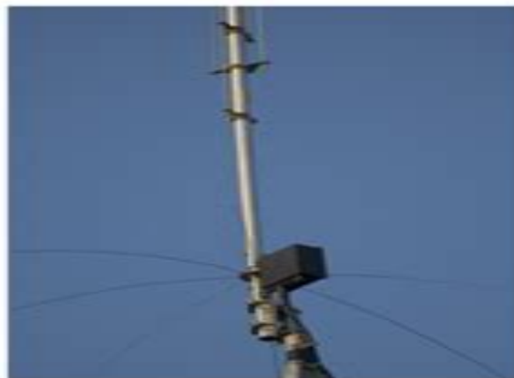
Matching network and base of stubs
