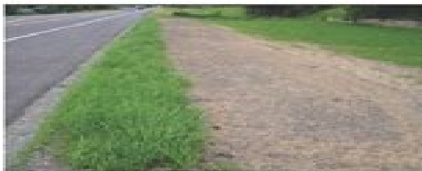
Media Filter Drain Along SR 14 in Clark County, WA. Source: Washington State DOT, 2011.
