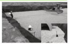
Place clean, crushed, angular stone foundation 230 mm (5") min. Install underdrains if required. Compact to achieve a flat surface.
