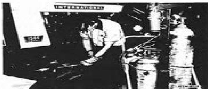
10. When using an acetylene torch always wear welding goggles and gloves. Keep a "charged" fire extinguisher within reach. Be sure the acetylene and oxygen tanks are separated by a metal shield and are chained to the cart. Do not weld or heat areas near fuel tanks or fuel lines and utilize proper shielding around hydraulic lines.
