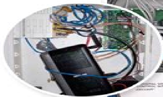
Above: wiring system cobbled together by non-certified installer. Right: structured wiring cabinet installed by certified professional.
