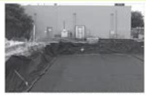
Place non-woven geotextile over prepared soils and up excavation walls.
