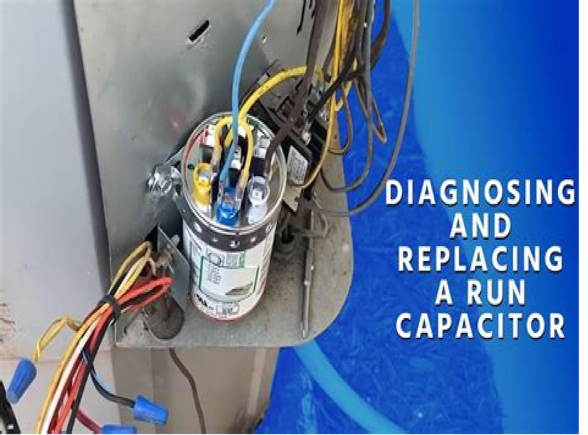
A photograph showing an electrical control panel with a run capacitor being replaced. The capacitor is a cylindrical component with a label, mounted on a metal plate. It is surrounded by various colored wires (yellow, blue, red, black) and other electrical components. The background is a blue wall.
