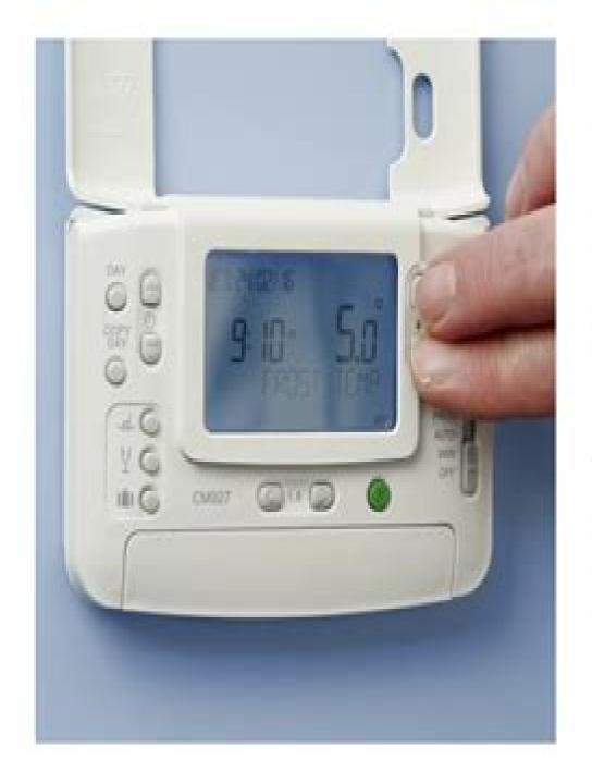
Step 1 Move the Slider into the Off position
