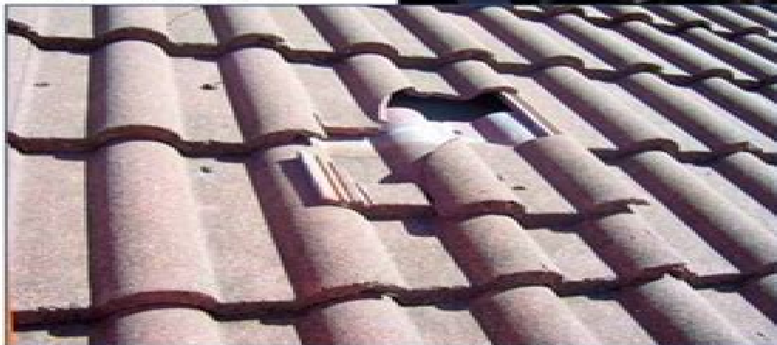
Photo 6 – Damage to concrete tile.
